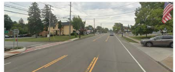
EXISTING CONDITIONS PHOTO. JULY 2022 (INTERSECTION AT N. BUFFALO ST. & SUNSET TERRACE)
